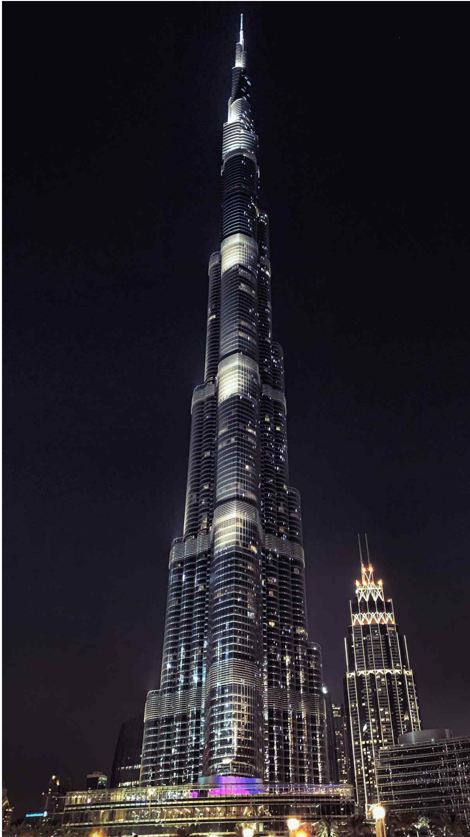
Fig. 1.1.: The Burj Khalifa. Based on the Hymenocallis Flower, the Burj Khalifa has three 'wings' which surface area progressively gets smaller as the building gets higher. As the cross-section of the building changes, this affects the wind flow and disrupts resonance from occurring. Picture taken by Shahin Ghanbari.
